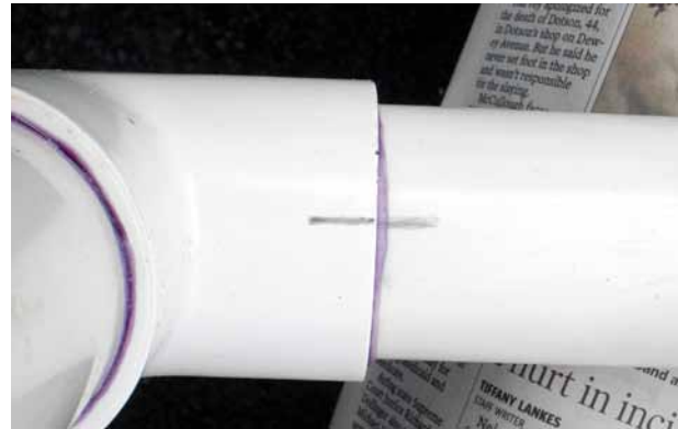
Figure 13: Line the marks up before the glue sets.
