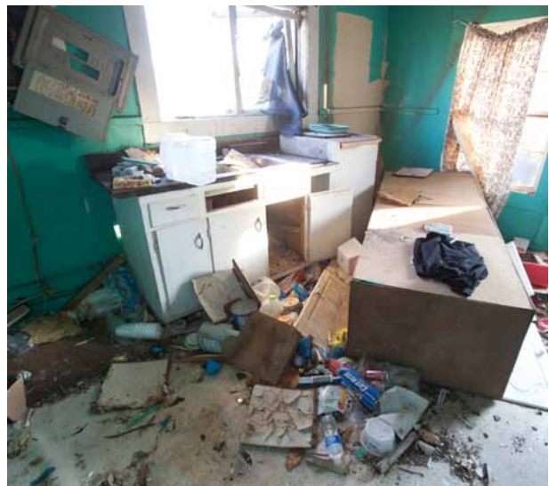
Even now, a year after the tornado hit, Hackleburg is still in the process of rebuilding.
