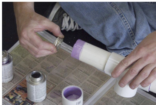
Read the directions for primer and glue carefully. You definitely want a good bond.
