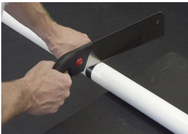
Above: Fine tooth hack saw makes easy work of cutting the pipe.
