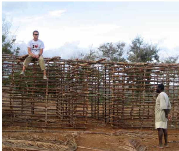
The house is framed and ready for mudding.
