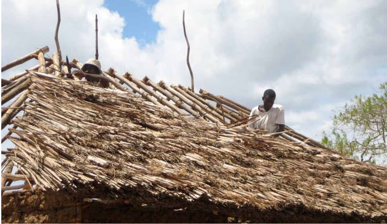
Constructing a watertight roof entirely from materials growing nearby.
