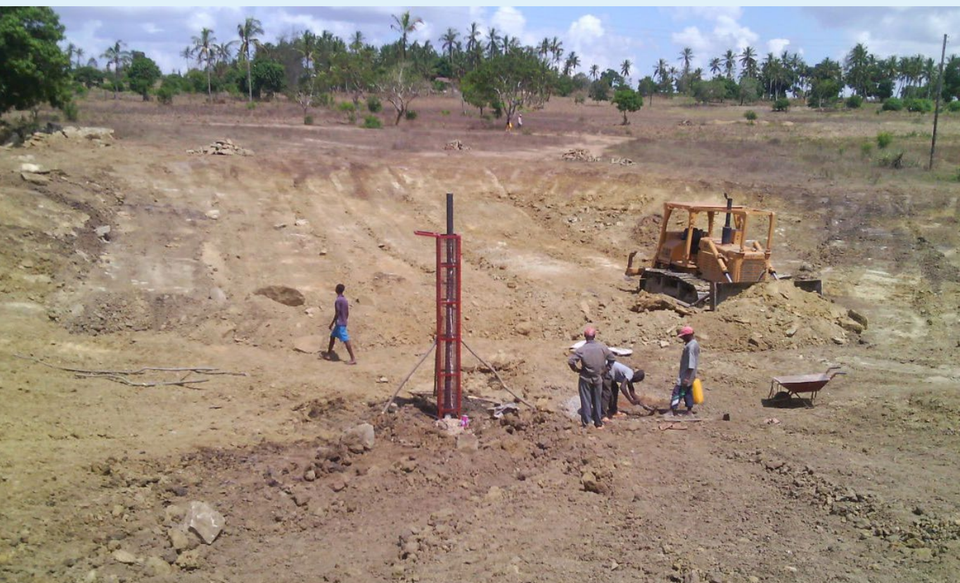
Aside from this filtration pipe, the entire dam is constructed with earth.
