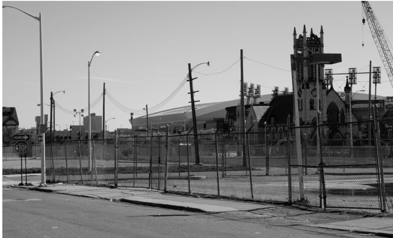
Construction crews are part of the Detroit skyline throughout downtown and its Midtown neighborhood. The city's core is becoming vibrant, while the remainder continues to decline.
