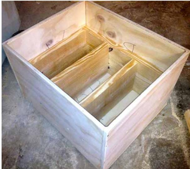
***Drive several screws through the plywood and inside the inner frame to secure it.***
