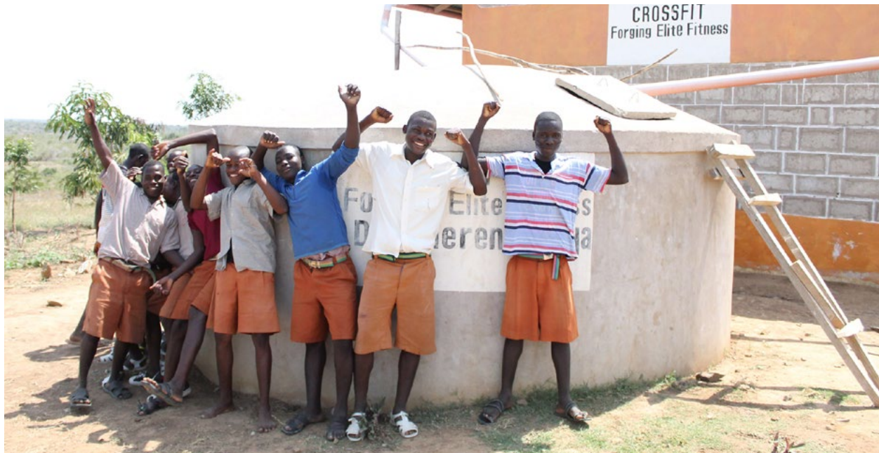
With a cistern collecting rainwater, students at the CrossFit school in Dzendereni can be assured of clean drinking water.
